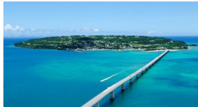
Bridge connected to Kouri Island
